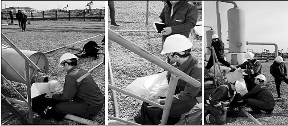
Actual images of the calibrated volume bag being used to measure the gas leak rate (from a stem packing valve prior to an associated gas liquid knock-out separator at the Bibiheybatneft OGPD)
