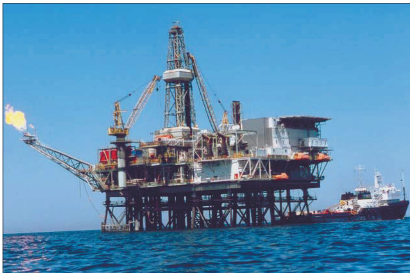
“Shah Deniz” gas and condensate field in the Republic of Azerbaijan
